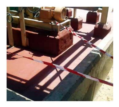
Belzona 4131 (Magma-Screed) is a two-component system for the repair and resurfacing of concrete and stonework.
